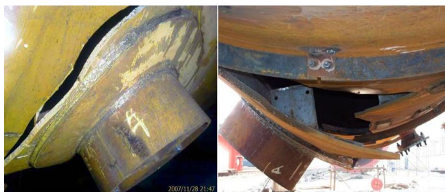
Figure 3 - Failure Pictures of Pressure vessels
